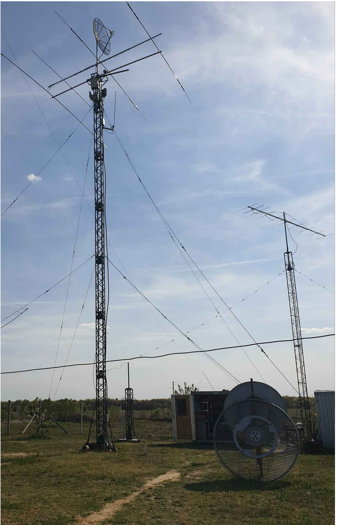
...and the antennas outside.
